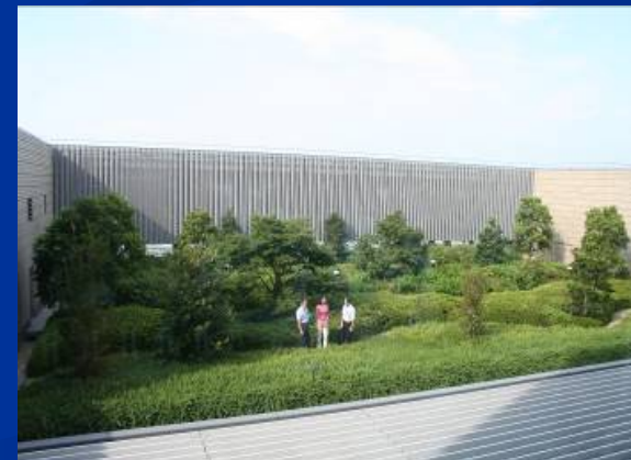
Head Office : Roof garden of 70m in height
